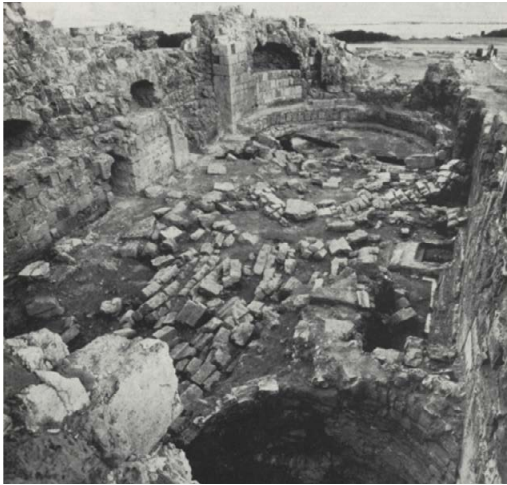
Fig. 7 – The Salmis central calidarium interior space after the last excavations with the fallen vault voussoirs still in situ (Karageorgis 1963).
