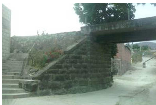
Fig. 6 – A railway bridge is incorporated into the contemporary architectural design leading to its preservation in absence of professionals. Note the concrete plaque added for pedestrian use. Source: the authors.
