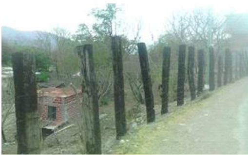
Fig. 4 – Railway material has been transformed in a fence, at the same time clearing the former railroad, creating an even surface to walk. Source: the authors.
