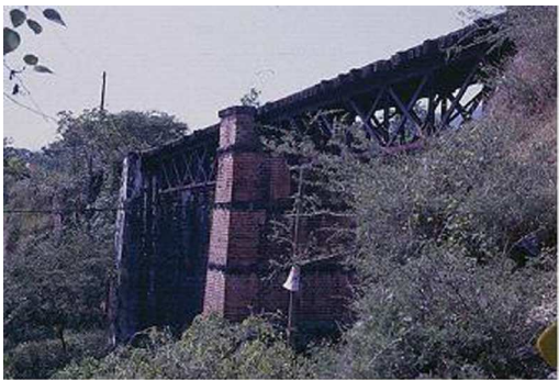
Fig. 2 – Bridge 1. A major structural work saving a 48 meters long cliff. Note the differences between the Northern pillar made of brick and the southern one built with gray concrete. Source: the authors.
