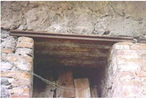
Fig. 8 – Rails used to form a lintel at the small fortress adjacent to the study area. Diversity of recycled materials can be observed in this constructive system. Source: the authors.
