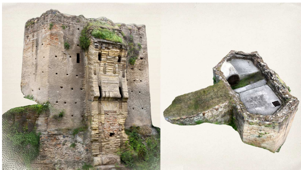
Fig.12 – Digital model produced by photogrammetry: Perspective view with the full texture.
